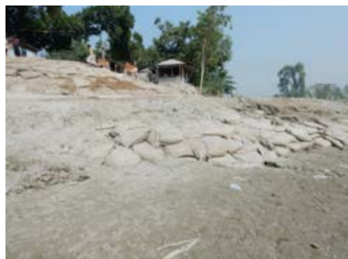
Figure 4.2: Sandbags for preventing erosion (Fulchhari, Gaibandha in Dec. 2014)
